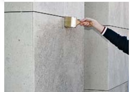
Re-application of ISOGRAFF, sacrificial anti-graffiti protective coating
