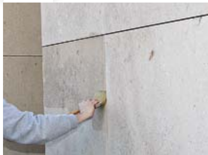
Application of ISOGRAFF, sacrificial anti-graffiti protective coating
