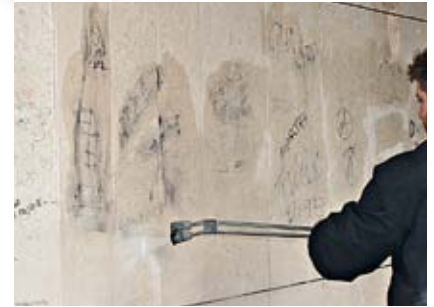
Removal of the defacing using a wire brush and/or pressurized hot water
