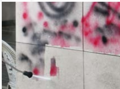
Simple removal of the graffiti with low pressure hot water
